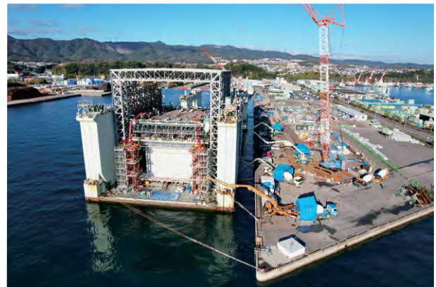
Photo-1 Offshore construction conditions
