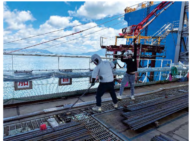
Photo-6 Supplying rebar from the upper level to the middle level
