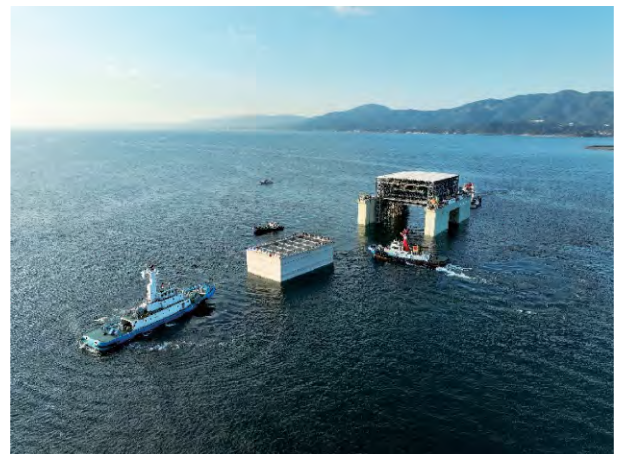
Photo-8 Caisson tow-out
